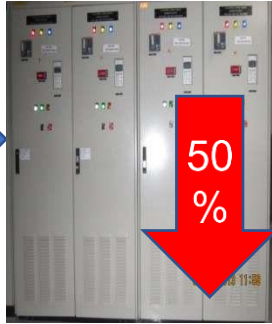
After: Installed 22 No's VFD s for all the bag filter fans
