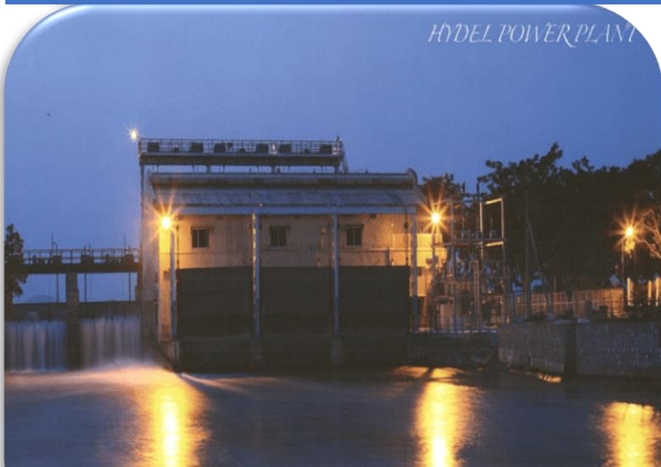
HYDEL POWER PLANT, NEKARIKALLU – 8.25 MW
