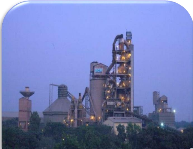
THE K C P LIMITED, CEMENT UNIT-I MACHERLA – 0.8 MTPA
