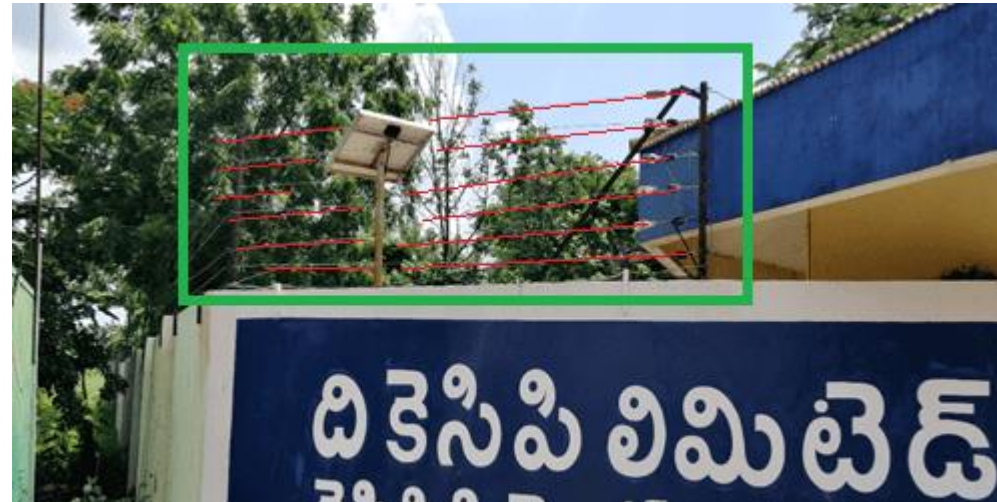
Solar Fencing around the Residential Colony
